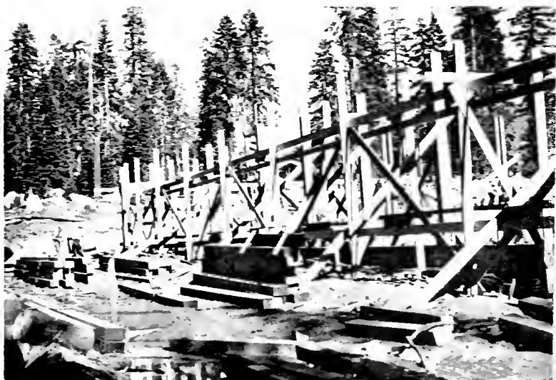
Truck shed framing being erected, Sept. 30
